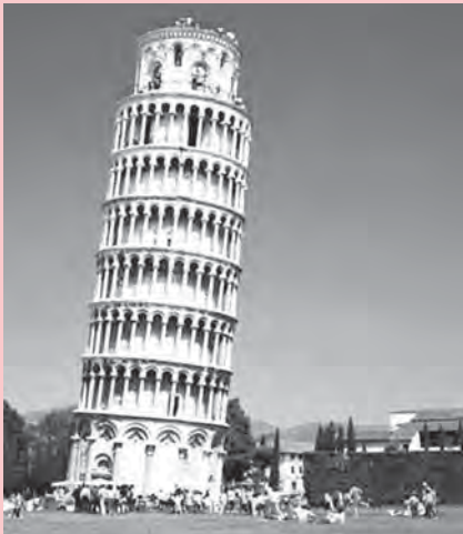
Leaning Tower of Pisa
